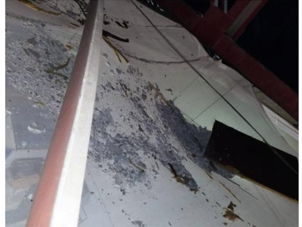
View of debris captured in the netting and suspended cover solution above the Coliseum seating area.
